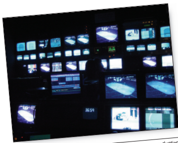
Figure 1.22 Production control compartment inside a large production truck. Slew of video monitors allow the director and others to see what each source is capturing. Sources are cameras, VTRs, graphics generation and effects devices, and outside sources such as other trucks. Computer monitors are increasingly present among the traditional video monitors as computers handle more of graphics effort and tracking of video and audio material.
