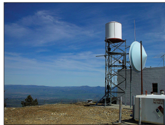
Figure 1.21 Often television stations will have multiple receive sites, either to enable multiple live shots at once or to allow microwave shoots from a larger geographical area. The water tank-looking structure is a "radome" protecting a steerable microwave receive dish. This site is atop Loma Prieta south of San Jose, CA.
