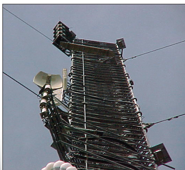
Figure 1.20 The receive end of the microwave path from the ENG truck. The dish just off picture center receives the microwave signal from the truck. The dish is steerable, which means it can be rotated in the direction of the ENG truck. As is the case here, these receive dishes are often mounted on the television station's transmit tower. There is usually a second microwave link to get the signal from the transmit site back to the studio.
